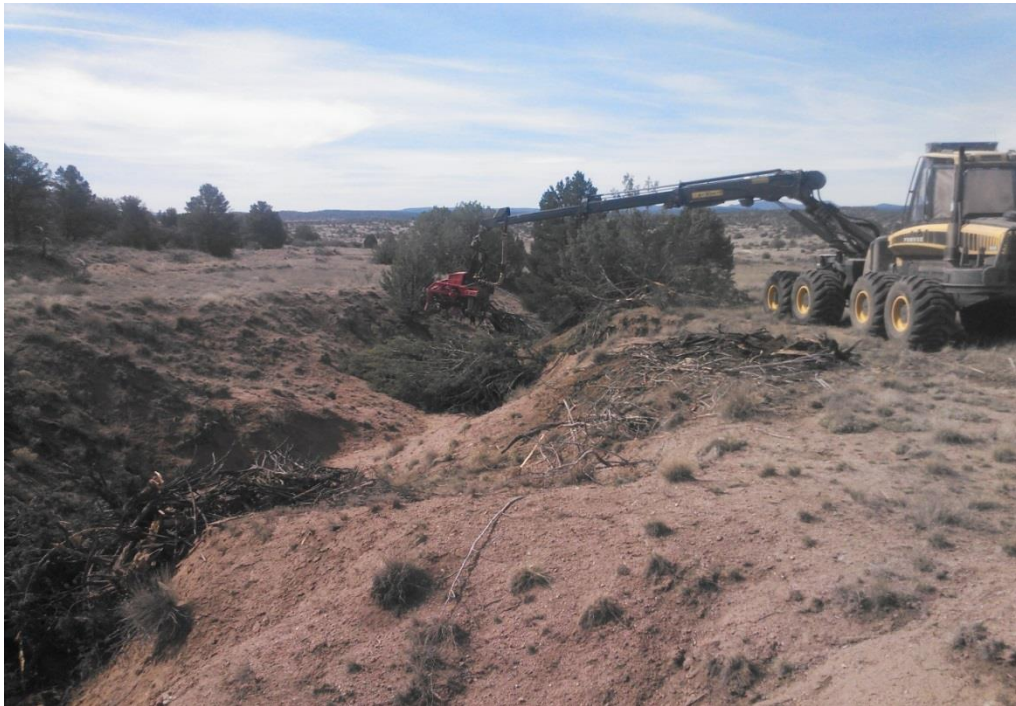
Figure 16. Picture of harvester placing juniper slash as an erosion control feature for silt dam. Note the ease of doing this work using the boom and shear head.
