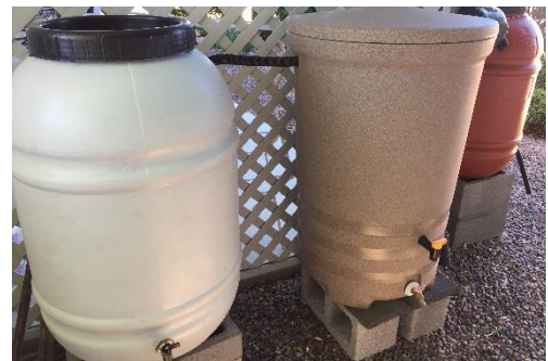
Fig 6 – Three rainbarrels fill from one downspout. Barrel on left was painted.
