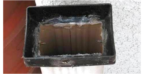
Fig 7 – Adapter connected to lower part of downspout. Note silicon seal .
