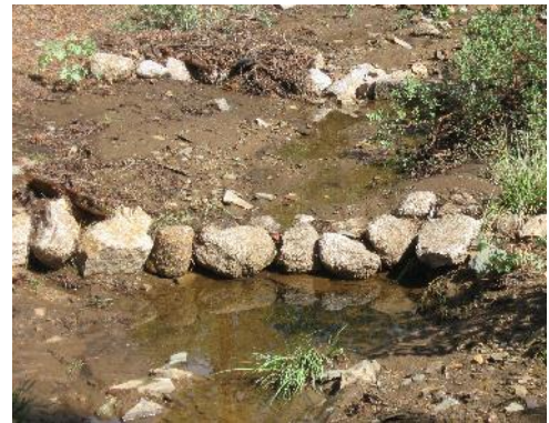
Fig 11 – Check dams in wash
