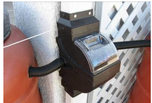
Fig 5 – Fiskars DiverterPro feeding two rainbarrels (since painted).
