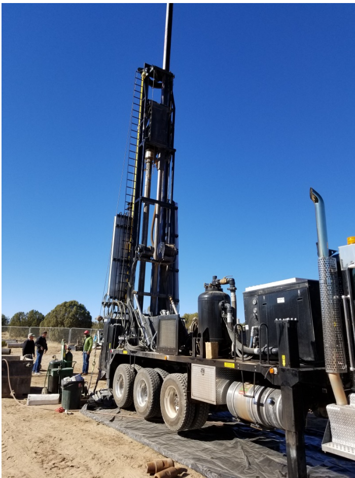
Drilling well MW-4d (March 4, 2018)
