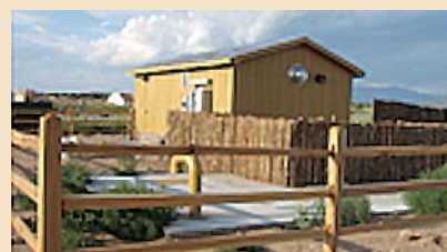
Esbr operations building.
