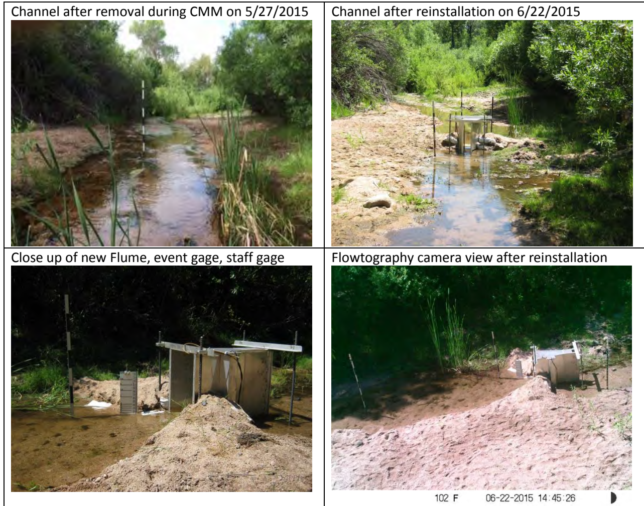
Figure 10 – Upper Walnut Creek Forest Service Flume Reinstallation
