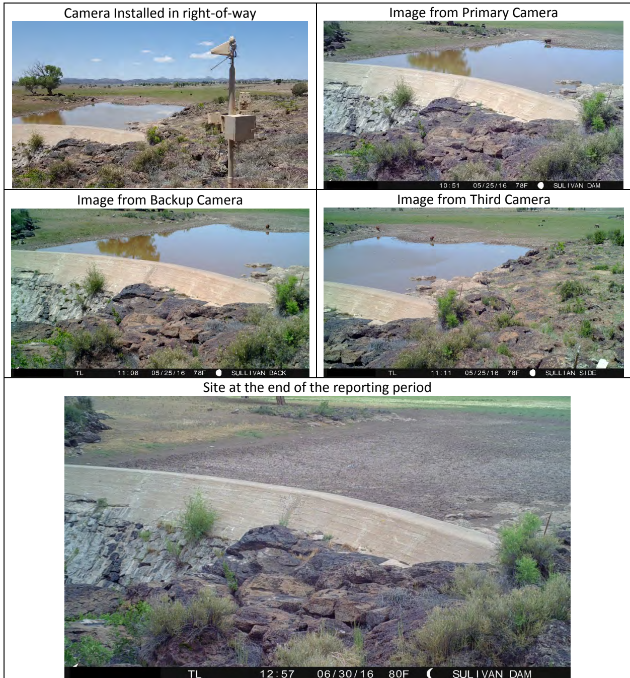
Figure 19: Sullivan Lake Dam SRP Flowtography® Camera Only Assembly Installation and Site Images
