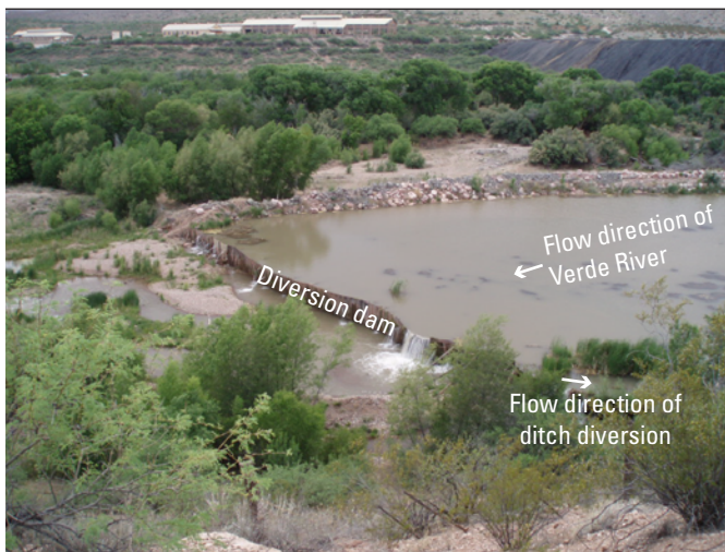
Figure 3. Surface-water diversion dam for Tavasci Ditch, Verde Valley, central Arizona. This dam allows water to divert by gravity flow into Pecks Lake and the Tavasci Ditch.
